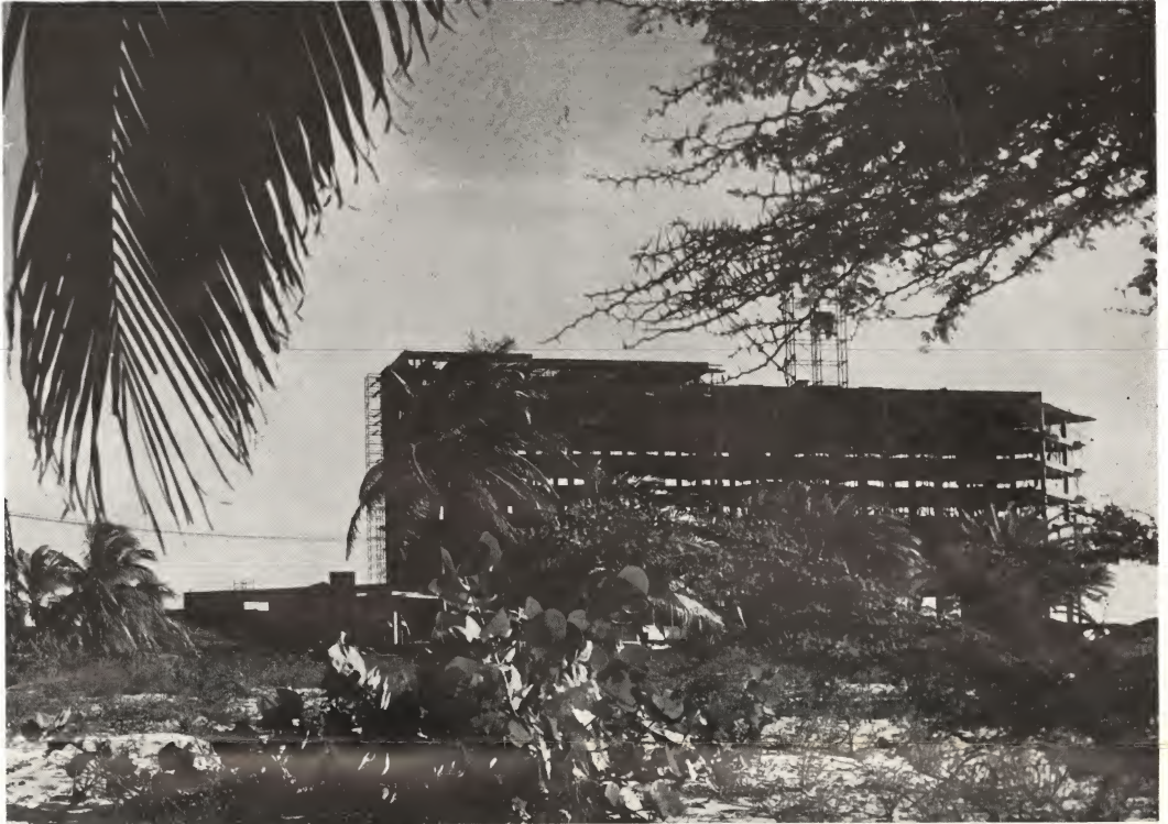
A view of the Hotel structure. All floors have been poured and Mr. J. Camping and his 400 men are working steadily, night and day, at the erection of the block partitions, the plastering and remaining finishings.
